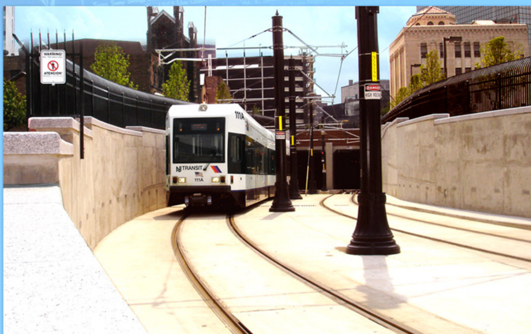
U-Wall Tunnel To At-Grade Transition
