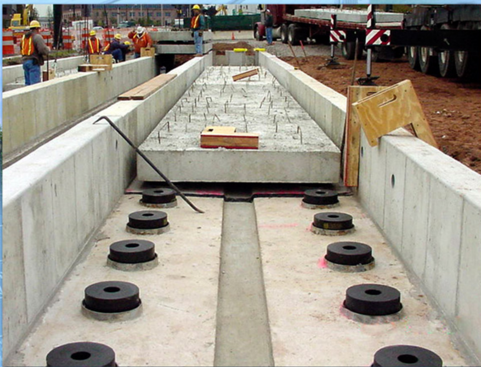
Floating Track Slab Construction
