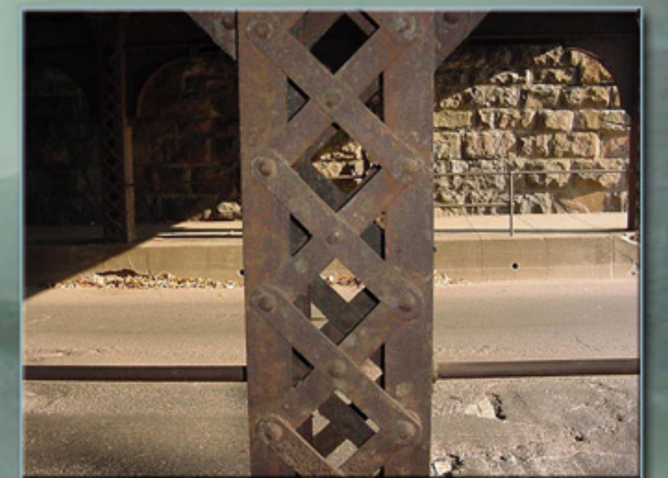
Original Lacing Bar
