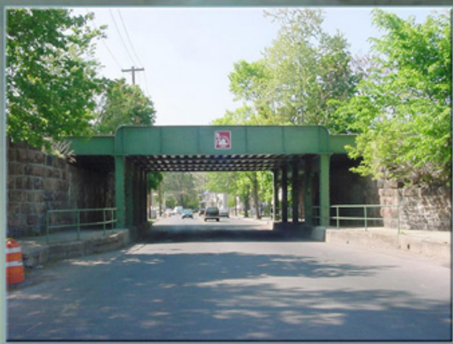
Restored Bridge Elevation
