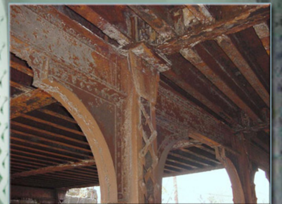
Top of Column Pre-restoration
