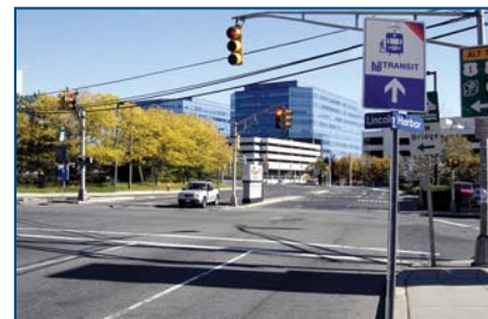
Traffic signal Improvements for 10 Intersections - Hudson County NJ
