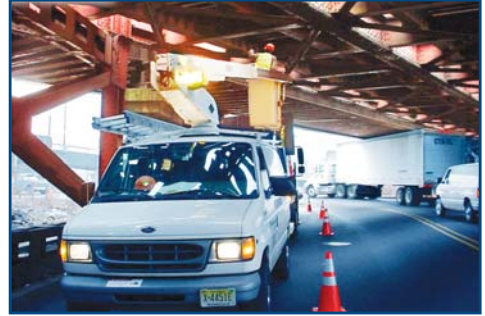
Undergrade Bridge Inspection - Morristown Line - NJ Transit
