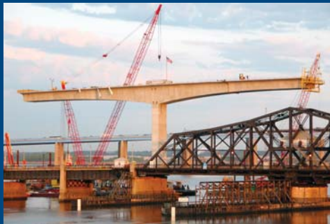
Construction Inspection - Victory Bridge, Route 35 NJDOT
