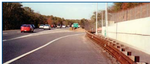
Garden State Parkway Interchange 77 - NJTA / Parkway Division
