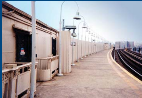
Civil Engineering - Sixteen Stations on White Plains Rd. Bronx - MTA / NYC Transit
