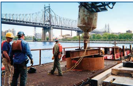
FDR Drive SB Reconstruction Construction Inspection - NYSDOT
