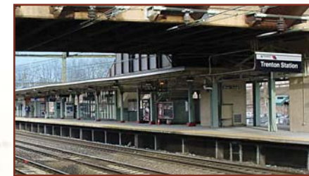
Construction Management for the Rehabilitation of Trenton Station - NJ Transit
