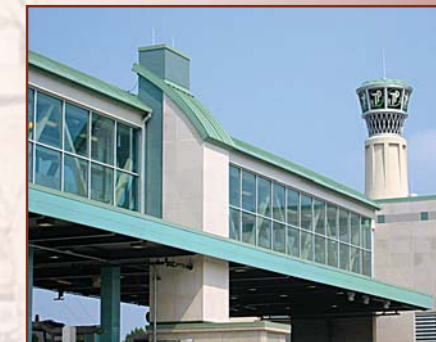
Construction Inspection for Interchange No. 1 Toll Plaza - NJTA
