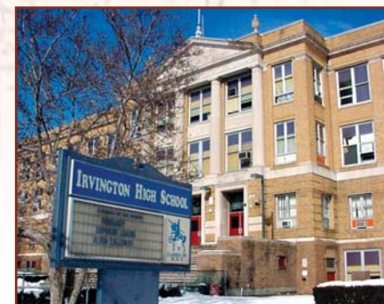
Construction Management of Irvington Township Schools - NJSCC
