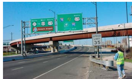
Inspection of over 600 Cantilever and Overhead Sign Structures - NJDOT - NYSDOT
