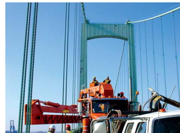
In-Depth Inspection & Deck Condition Assessment of the Walt Whitman Bridge Suspension and Anchorage Spans - Delaware River Port Authority
