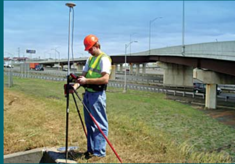
GIS Mapping and Inspection of over 4000 Drainage Outfalls on the Garden State Parkway & NJ Turnpike
