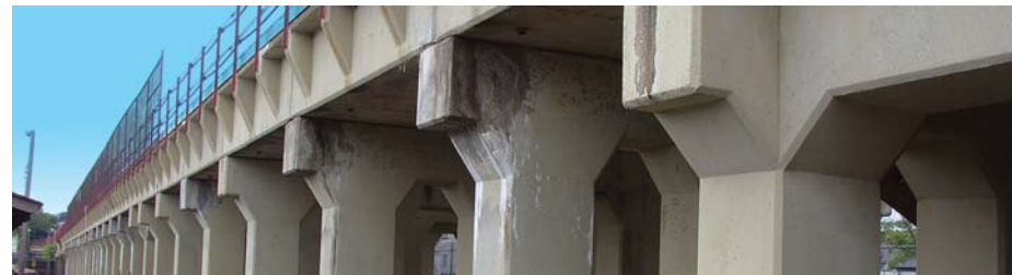
In-Depth Inspection of Bridges and Viaducts carrying Staten Island Rapid Transit - MTA / NYC Transit
