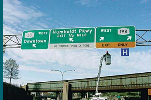
Inspection of over 300 Sign Structures in Region 11 & Upstate - NYSDOT (2003 - 2006)
