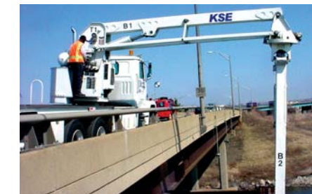
NBIS Inspection of over 300 Garden State Parkway Bridges - NJ Turnpike Authority
