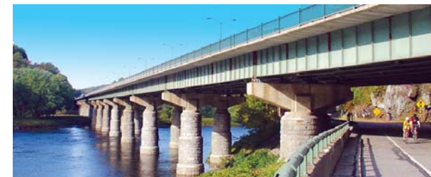
2005 Systemwide NBIS Substructure Inspection - Delaware River Joint Toll Bridge Commission
