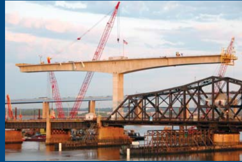
Construction Inspection - Victory Bridge, Route 35 NJDOT
