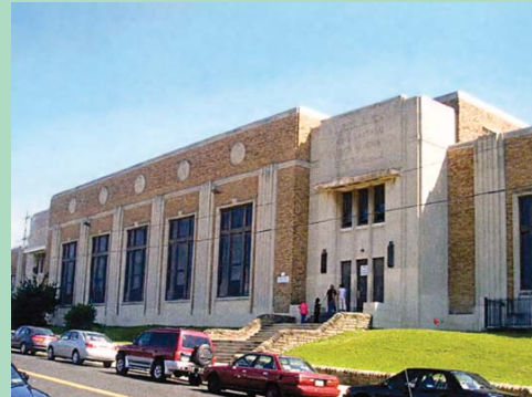
Bartram High School - Demolition & Roof Upgrade Philadelphia, PA
