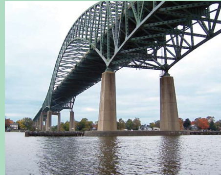
Delaware River Turnpike Bridge Rehabilitation Design, NJ-PA
