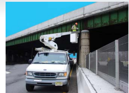
Biennial Inspection of Local & Arterial bridges in NY City & Upstate Regions - NYSDOT
