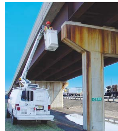
Bridge Inspection Program, Part B - NJ Turnpike Authority (2001, 2002, 2003, 2005, 2006)
